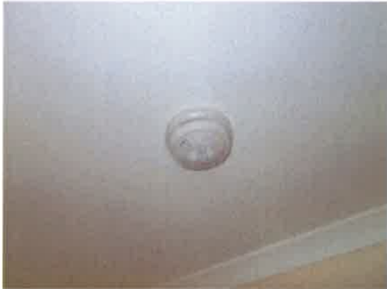
Kitchen - new ceiling mounted heat alarm
