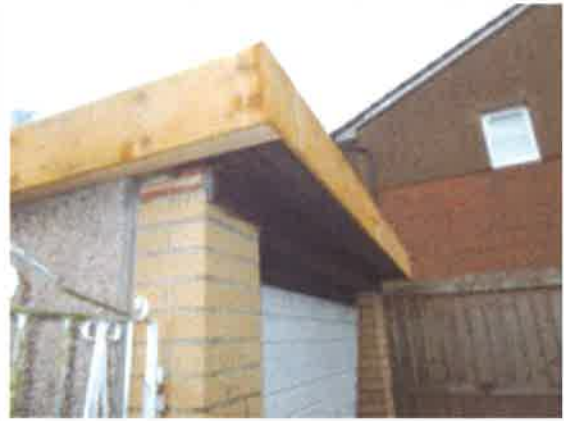
Garage - new fascia and soffit boards to side and front
