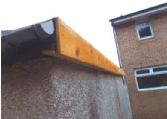
Garage - new soffit and fascia boards to left side
