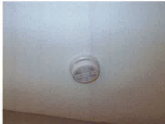
Living Room - new ceiling mounted smoke alarm
