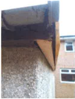
Garage - existing fascia and soffit to rear showing gaps and rot
