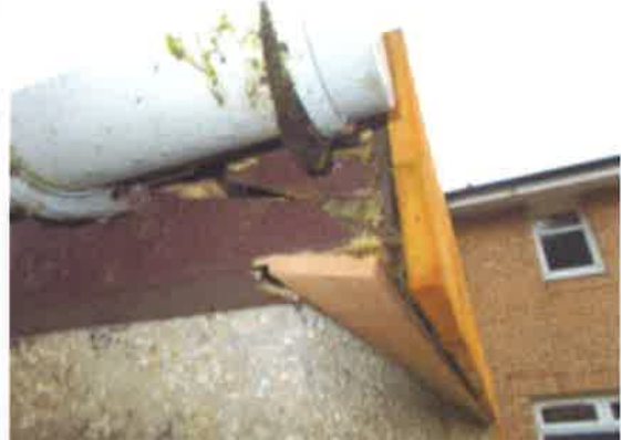
Garage - existing fascia and soffit to rear showing gaps and rot
