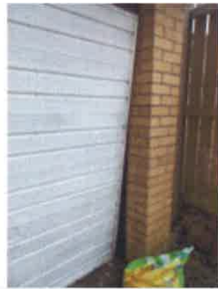
Garage - defective metal up and over door
