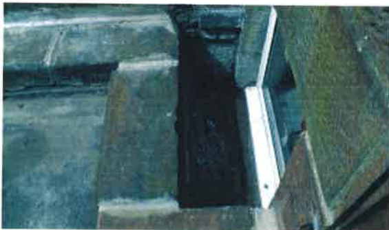
Photo 3 – External sill and soakaway
