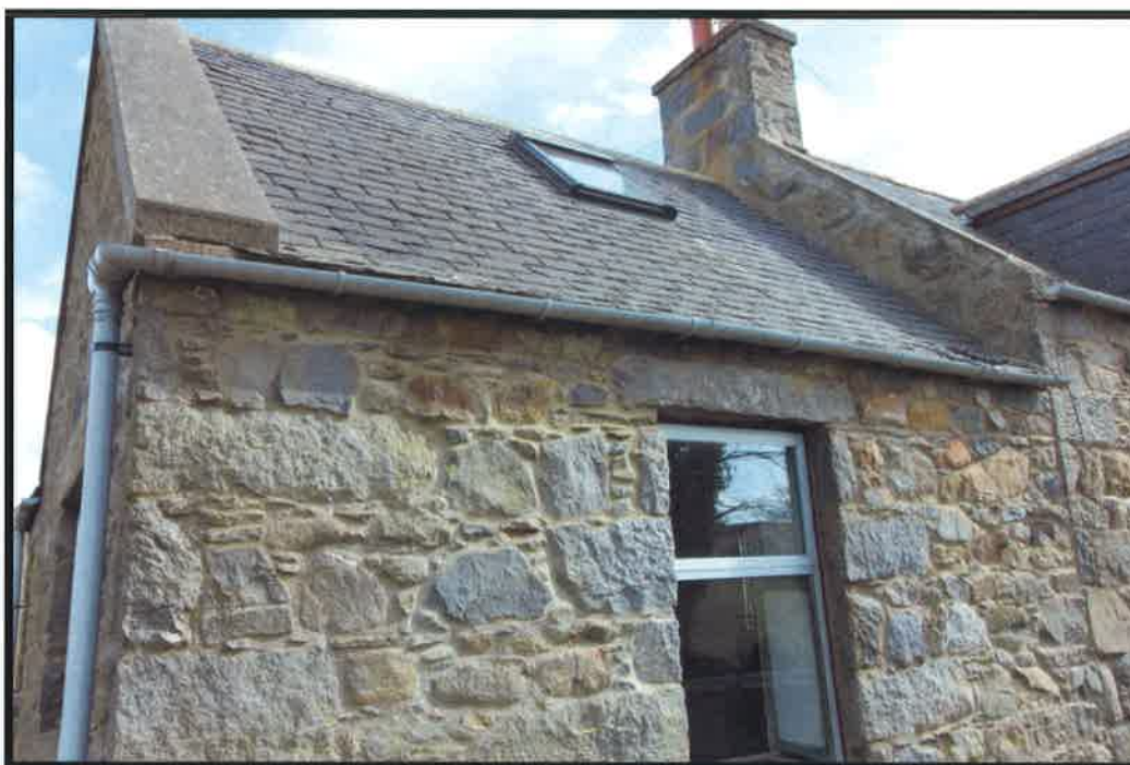
Figure 7 Front elevation left hand side gutter and downpipe - intact/secure.
