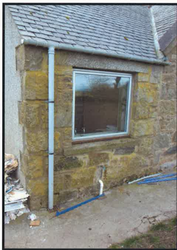
Figure 9 Left hand rear corner and downpipe - downpipe re-clipped.
