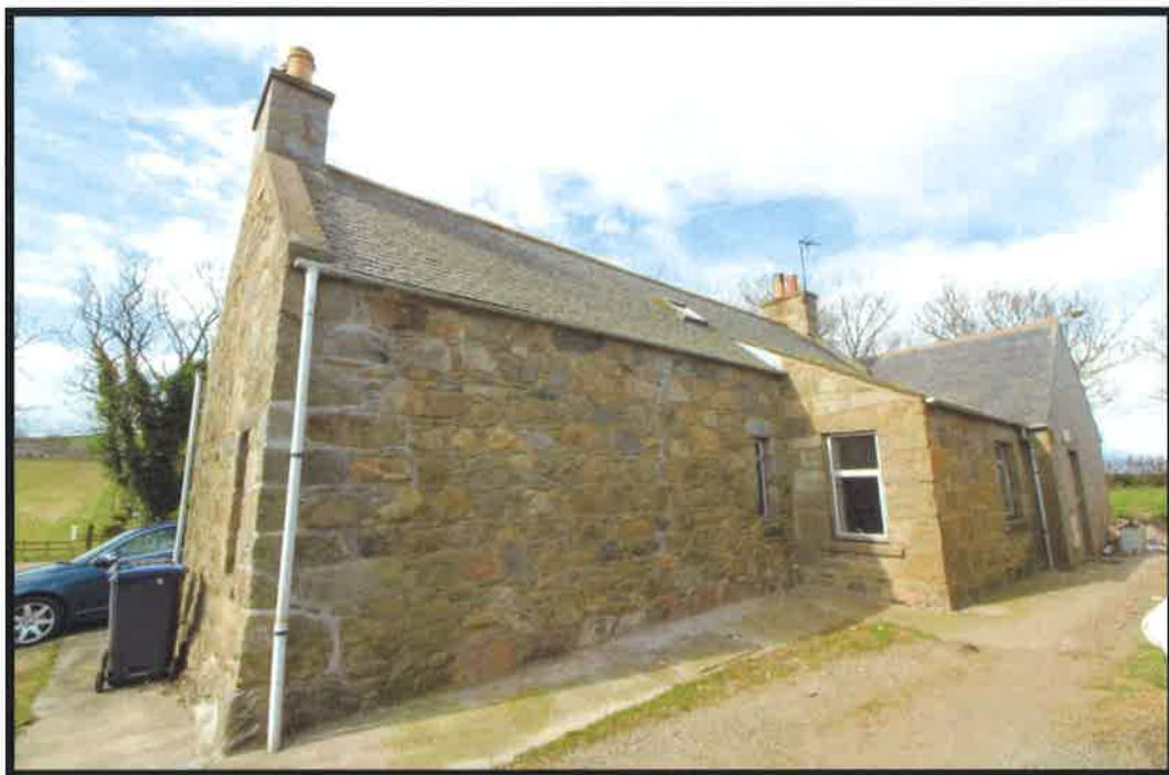
Figure 11- Rear left corner - both cracked areas re-pointed.
