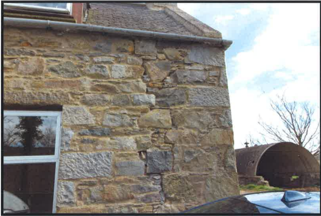
Figure 4 Front elevation right hand side vertical crack - raked out.
