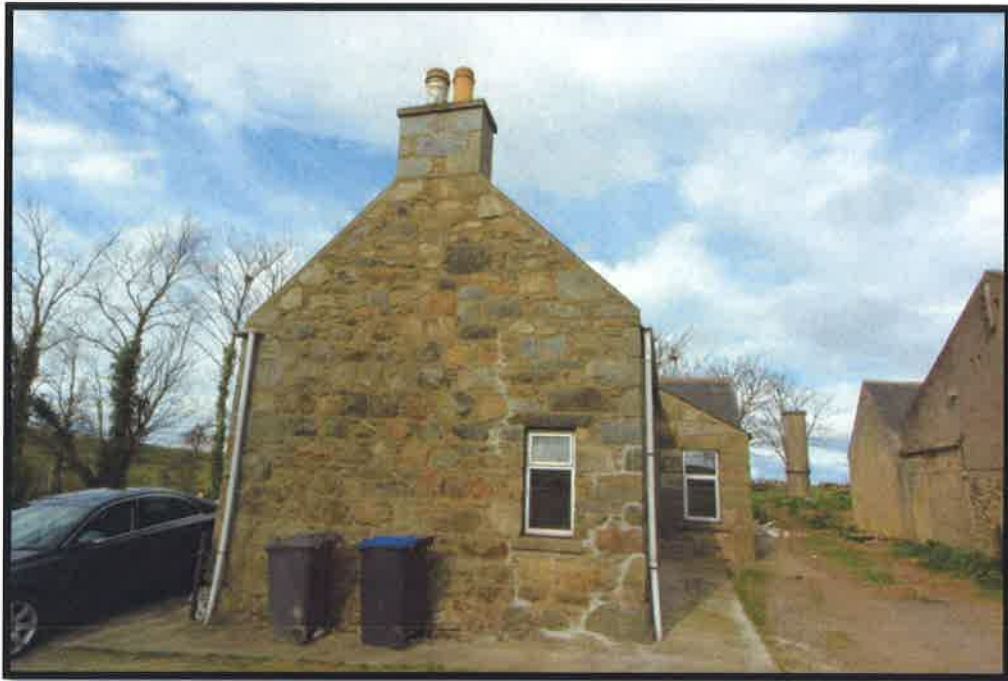
Figure 2 Right hand gable elevation - cracks re-pointed.
