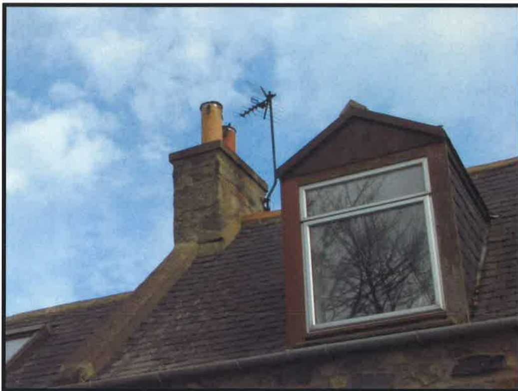
Figure 6 Left left hand chimney - cowls missing.
