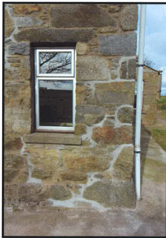
Figure 3 Right hand bedroom window - cracks re-pointed.
