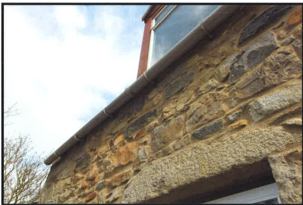
Figure 5 Front elevation left hand gutter - broken gutter clips.
