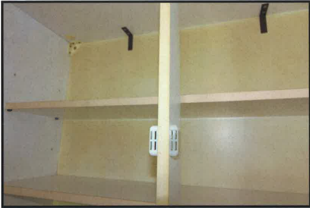
Figure 16 Wall units - catches fitted.
