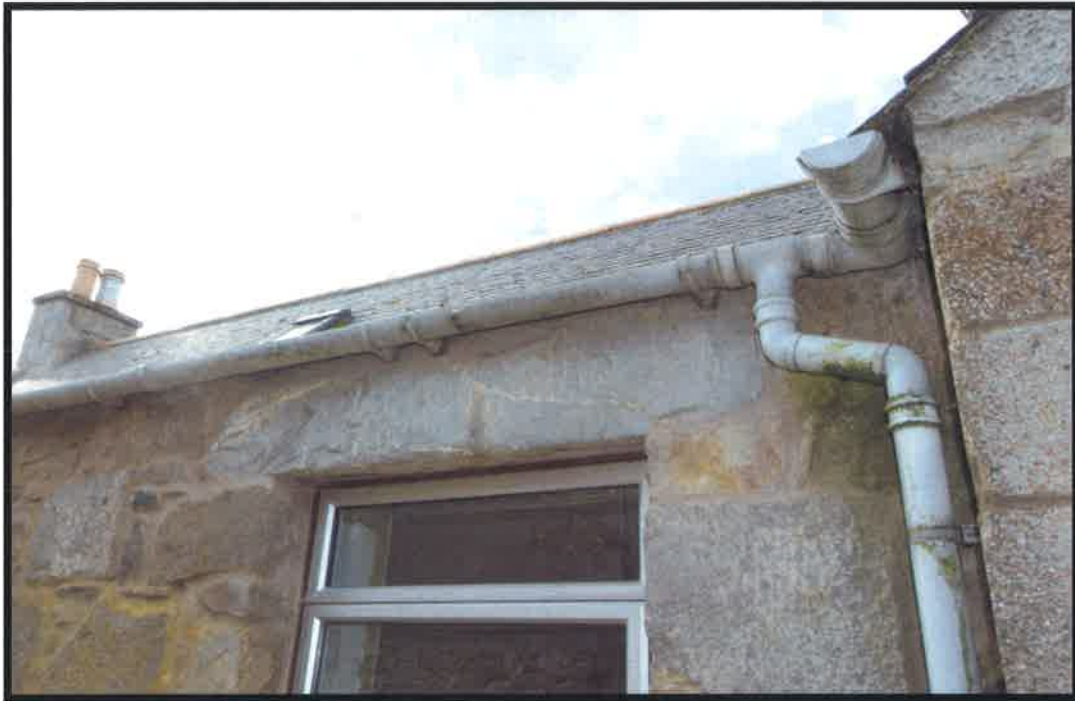
Figure 10 ~ rear elevation gutter - cracked as before, broken clips evident.
