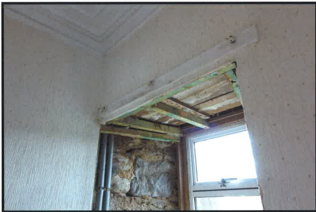
Figure 16 Ground floor bedroom window (typical window) - linings stripped out at ingoes
