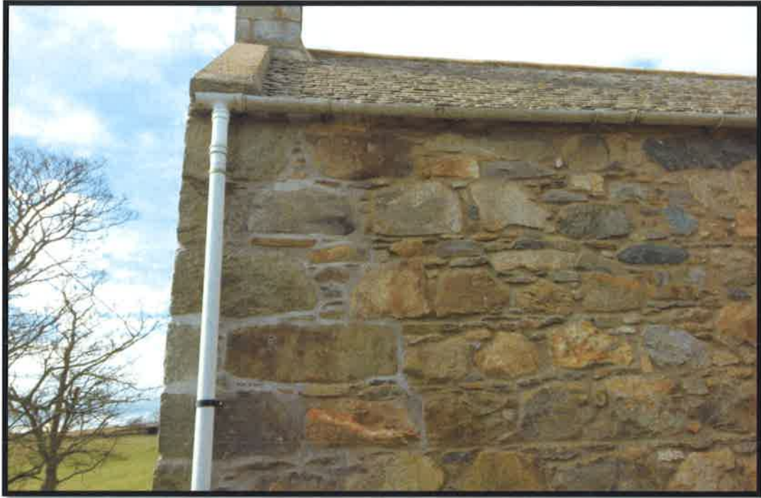
Figure 12 Rear left corner - crack re-pointed, downpipe re-clipped. Broken/missing gutter brackets.
