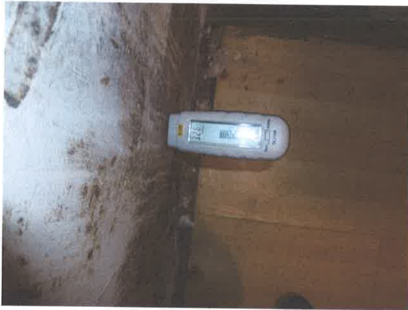
15. Moisture reading at pantry
