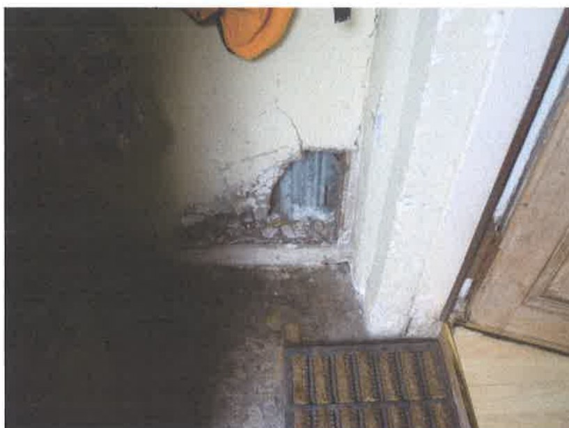
13. Damaged plaster at porch
