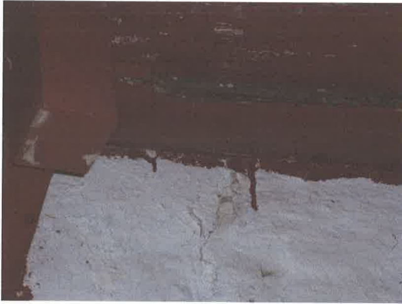
9. Gaps at eaves soffit
