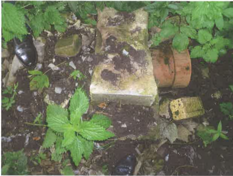
5. Septic tank outfall showing use of tenant's plant holder as termination
