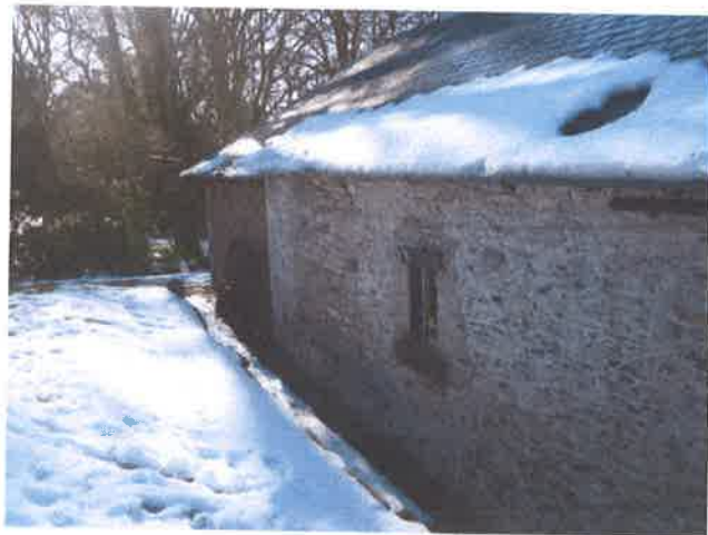
Render removed north-east elevation
