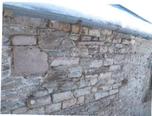
Pointing issues north-east elevation
