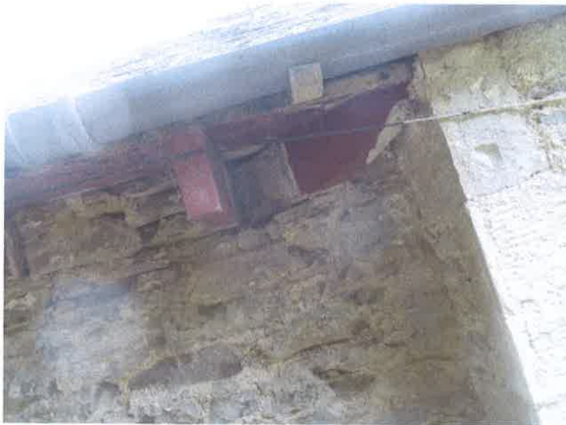
10. Holes at wallhead/ eaves soffit
