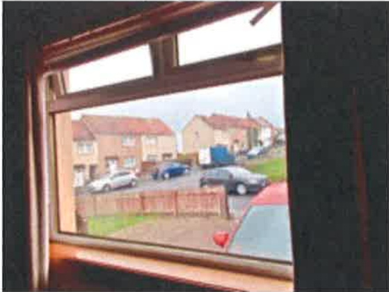
Living Room window - front
