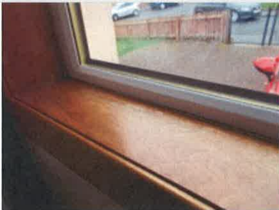
Living Room window - front
