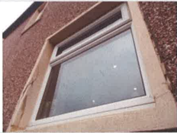
Kitchen window - external
