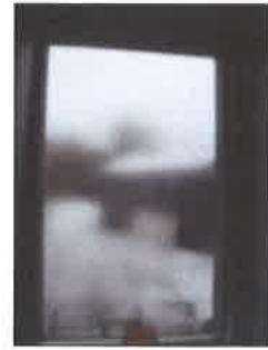
7. Hall landing window
