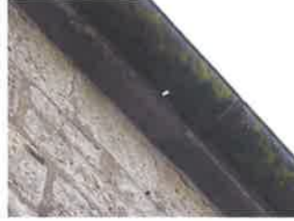
15. Eaves level gutter
