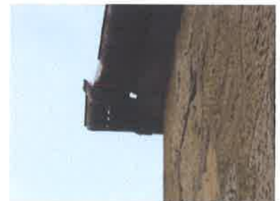
13. Eaves level gutter
