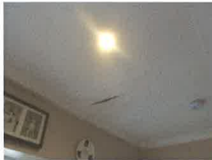
9. Water Damage Kitchen Ceiling
