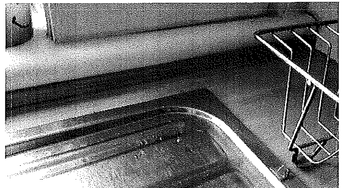
Photo 5: splashback to kitchen sink resealed
