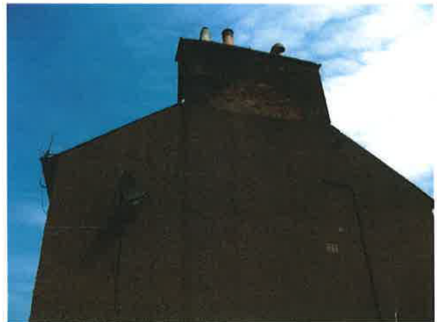
04 - Gable wall (roughcast except for chimney head)
