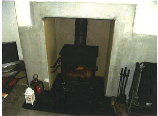
02 - New multi-fuel stove (with new back boiler)
