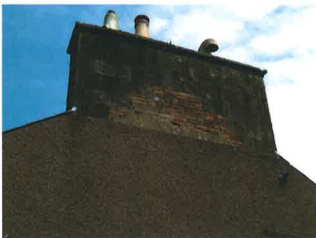
05 - Chimney head (part brick & part stone block)
