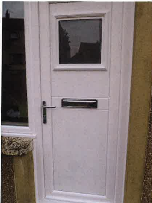
Replacement front door - June 2017
