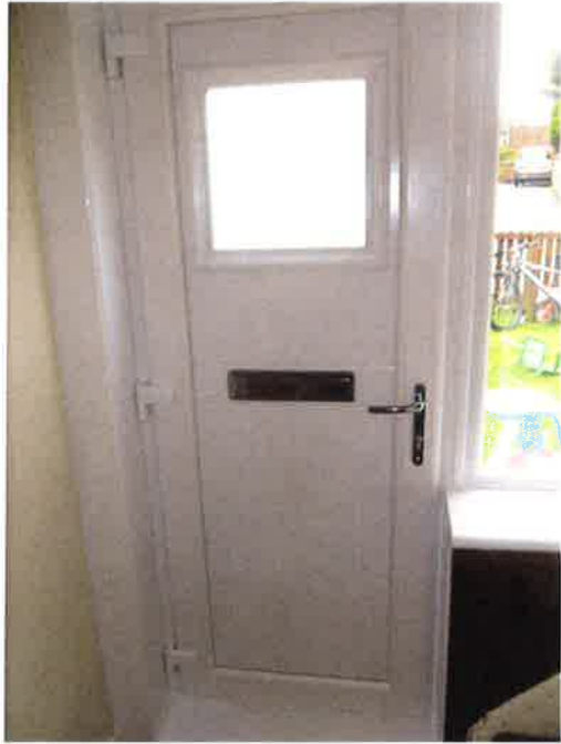
Replacement front door - June 2017
