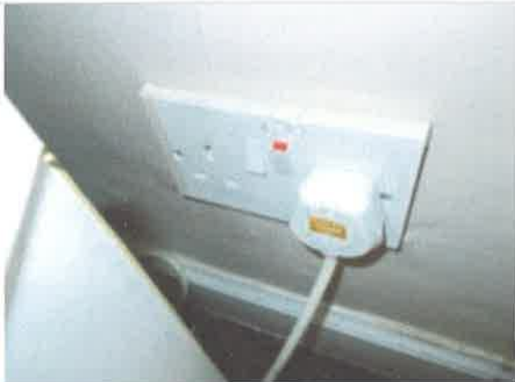
Double socket in Living Room - defective/jammed switch
