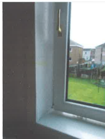
Back Bedroom window - restricted opening/loose frame and defective opening mechanism
