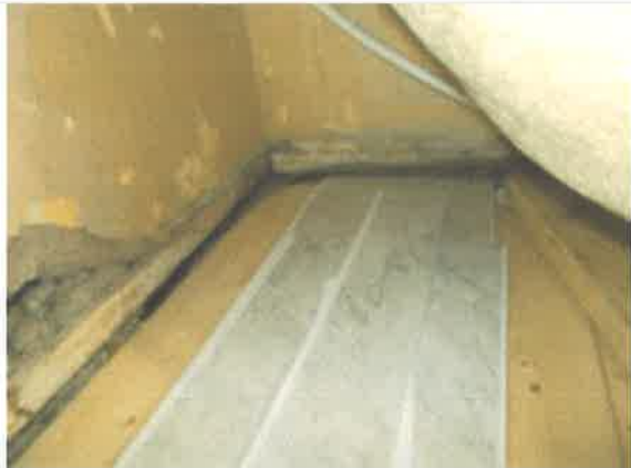
Bathroom - floor under bath - showing electric cable
