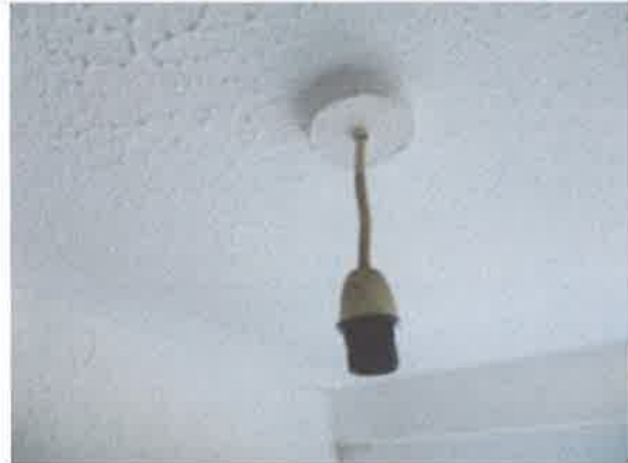
Light Fitting - ground floor hall ceiling - cracked/ loose cable
