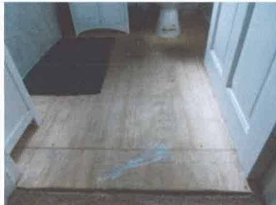
Bathroom floor - exposed plywood - no floor covering
