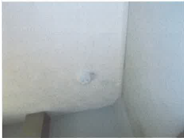
Ceiling mounted heat alarm - Kitchen
