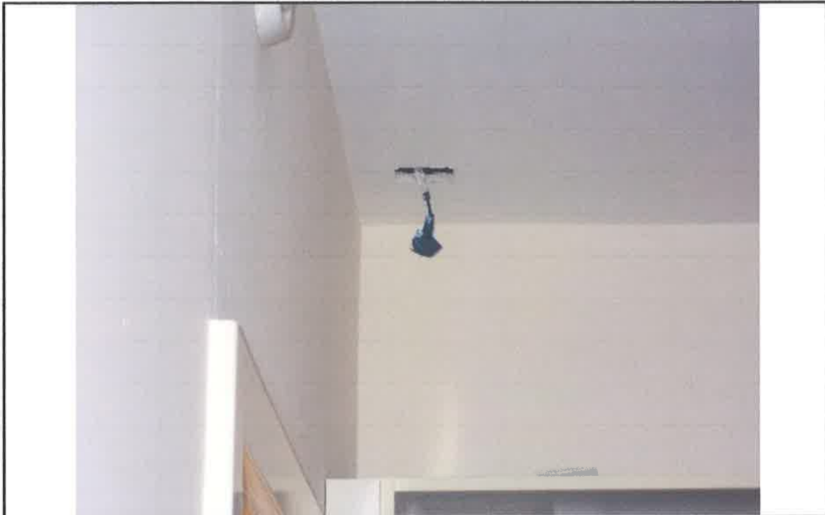
15. Loose cable hanging from hole in ceiling at Kitchen area of main living area
