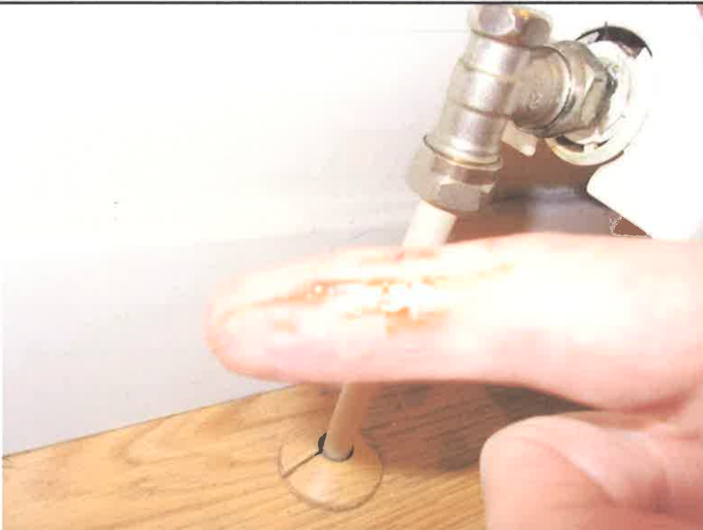
6. Liquid leaking from valve on other radiator in main living area
