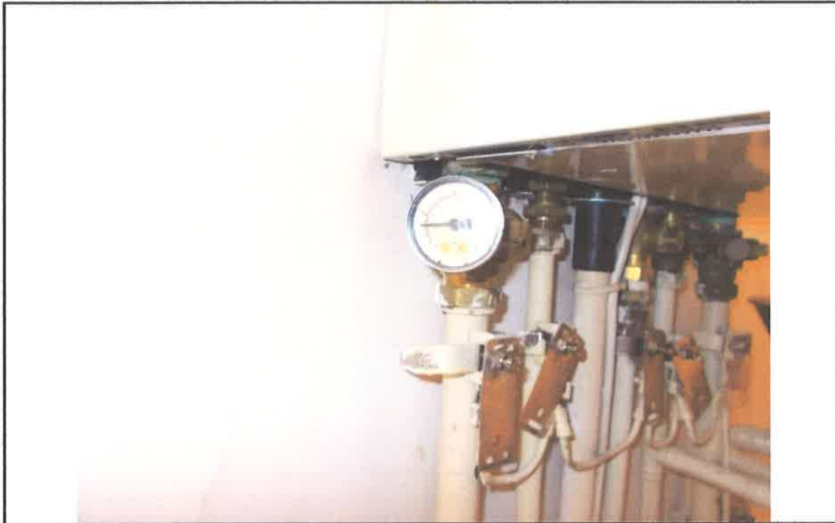
9. Pressure gauge on central heating system at boiler
