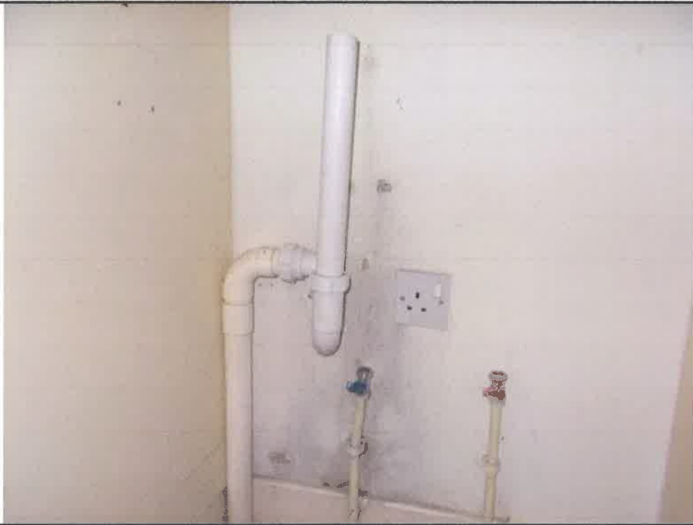
11. Supply and drainage pipework for washing machine
