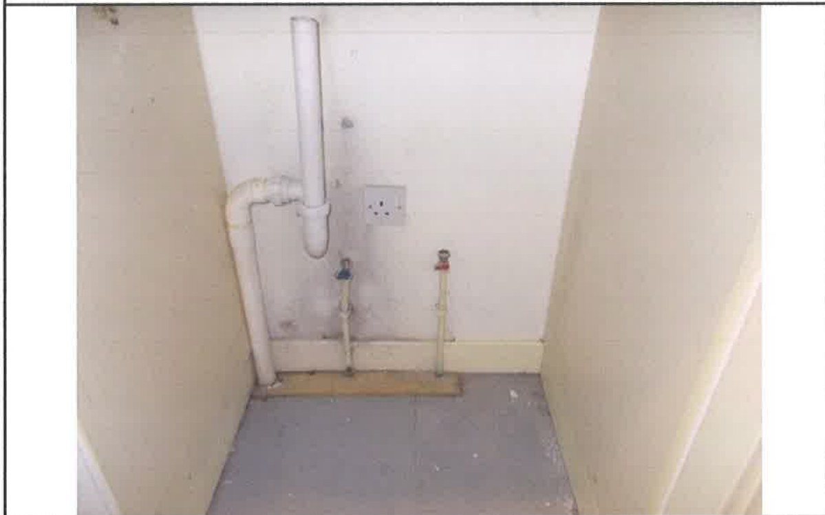
10. Supply and drainage pipework for washing machine
