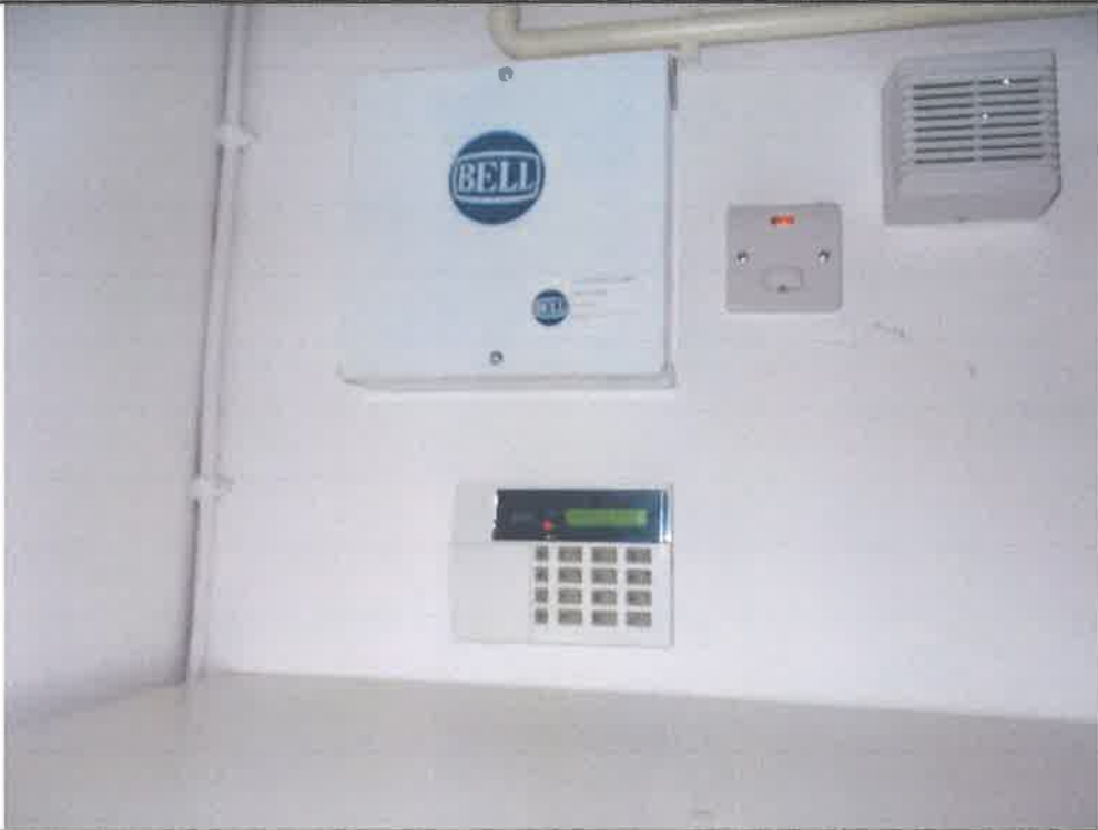
17. Intruder alarm control panel
