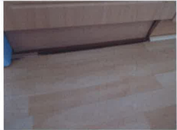
Kitchen - Floor adjacent to dishwasher
