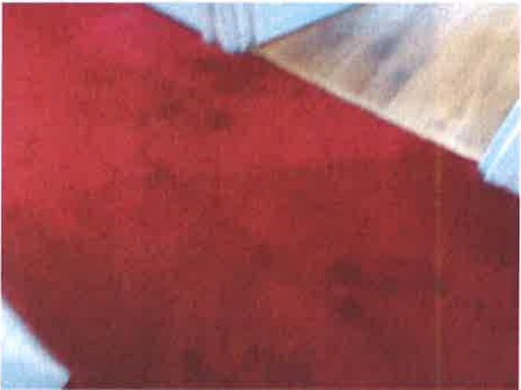
Landing floor - loose/damaged floorboard
