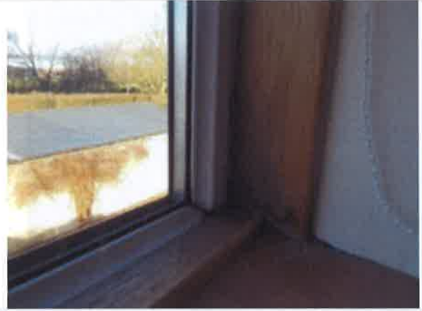
Master bedroom window - to rear
