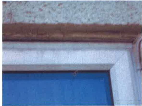
Living room window - external - gaps at top of window
