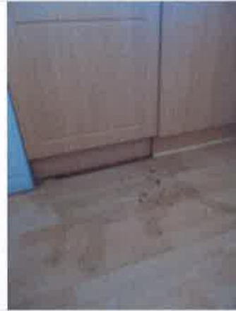
Kitchen - Dishwasher - showing flood from machine onto adjacent floor
