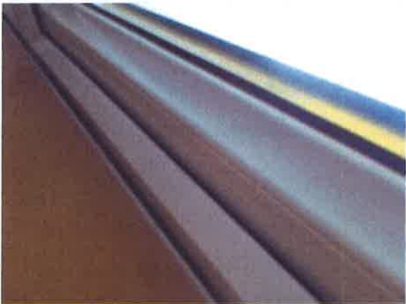
Living room window - gap at Silicon seal
