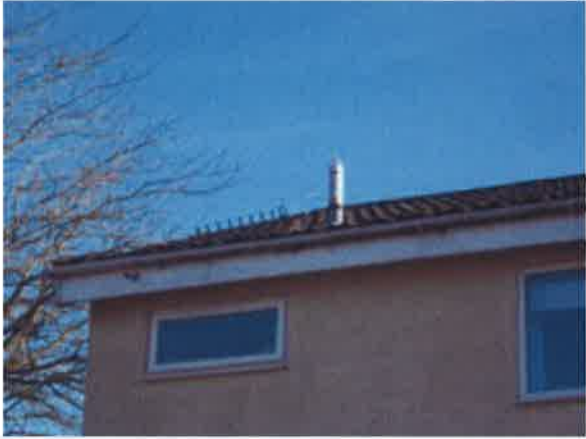
Television Aerial - lying unsecured on rear pitch of roof
