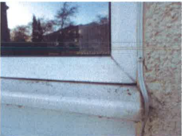
Living room window - external - gap at base of window
