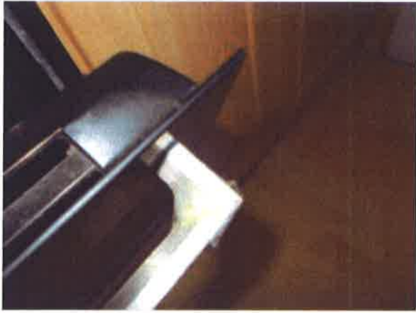
Kitchen - Oven door handle -secured with tape
