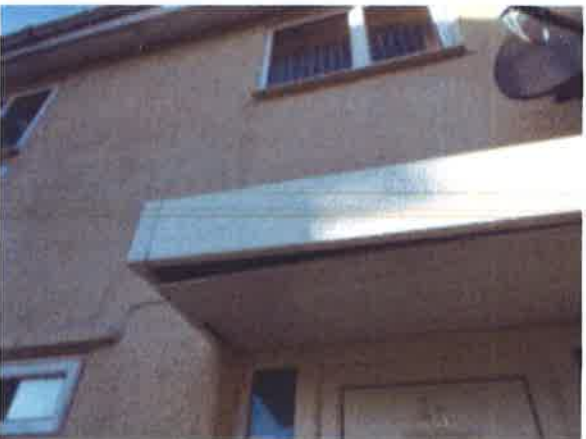
Canopy over front door - loose panel/gaps
