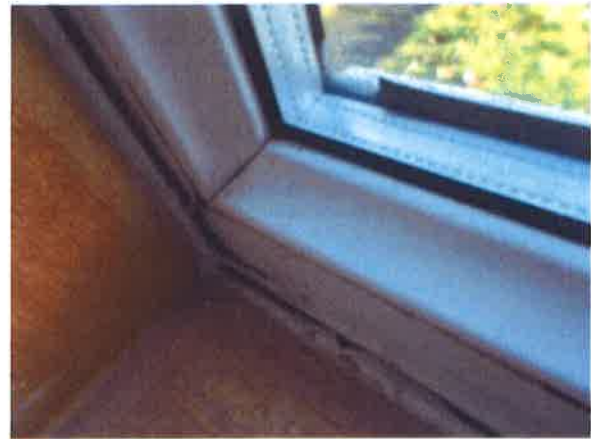
Living room window - gap in internal seal and Silicon seal to sill defective
