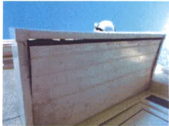
Canopy over front door - loose panel/gaps
