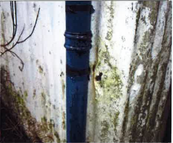
Photo 4 - Defective downpipe
