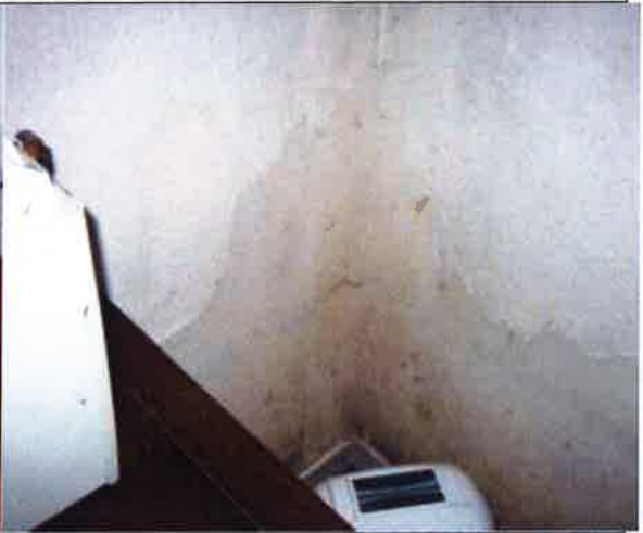
Photo 12 – Damp internally
