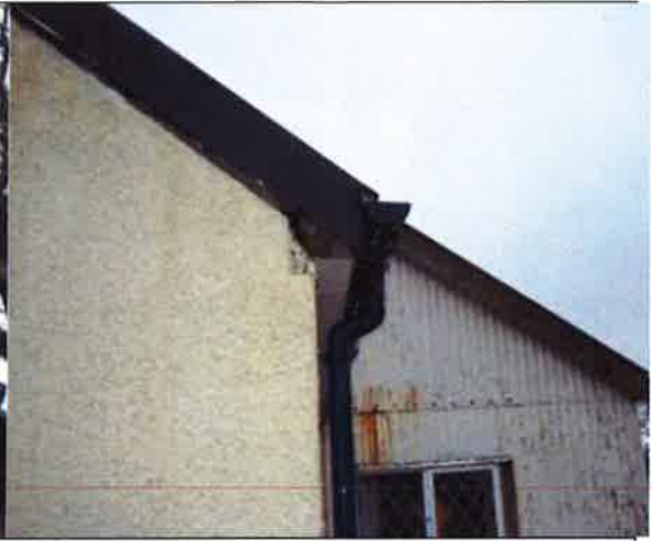
Photo 6 – Kitchen trim (at roof)
