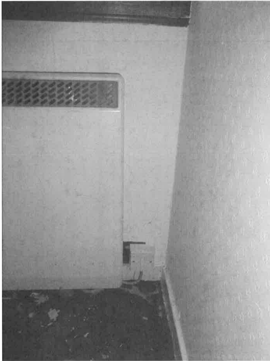
Night Storage heaters – being re-wired January 2017
