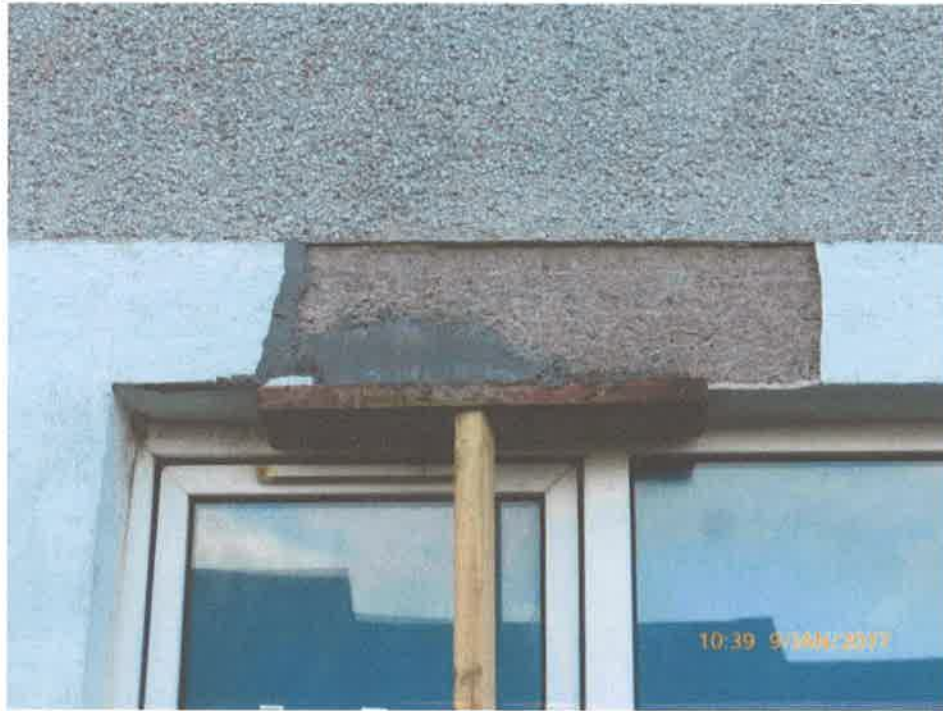
Detail of the repair being carried out above the living-room window
