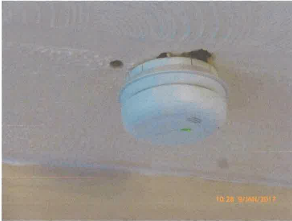
Holes in the ceiling around the new smoke detector
