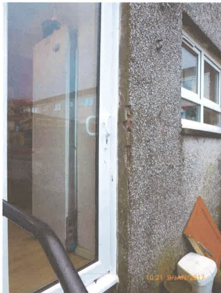
Cracked render outside the patio door
