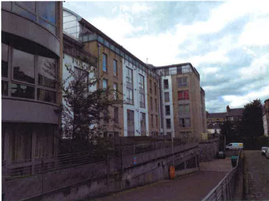
Rear of the building
