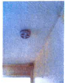
13. Hard wired smoke detector
