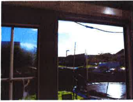
5. Patio Door at lounge
