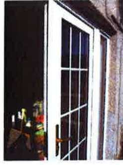
6. Patio door at lounge.
