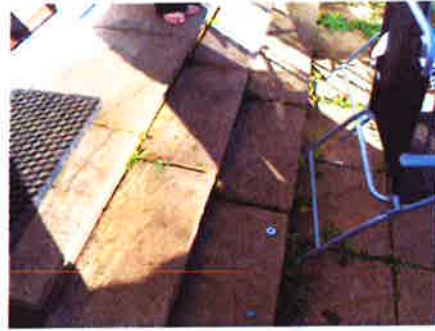
9. Steps at patio door
