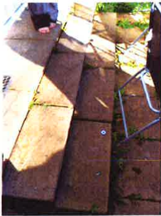
8. Steps at patio door
