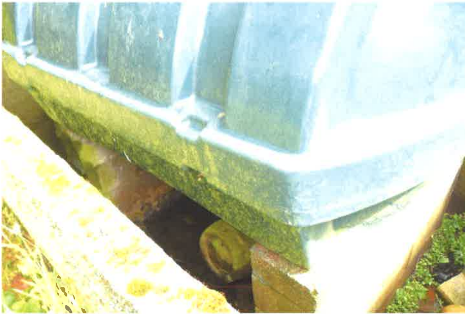
Oil tank supported on 2 piers.
