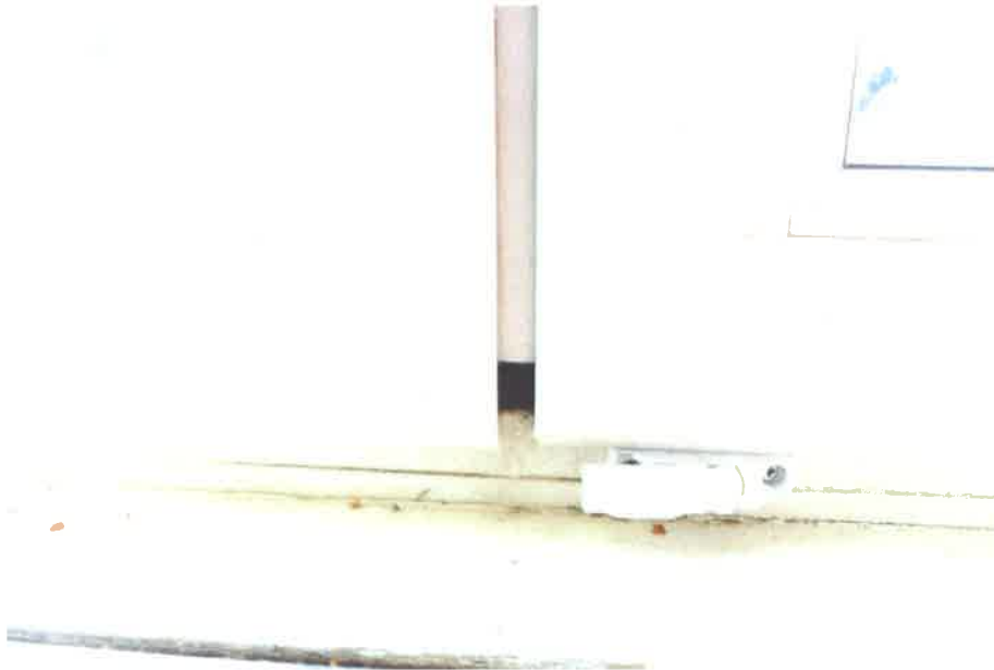
Bottom of Kitchen door showing gap at base and clip on right hand door.
