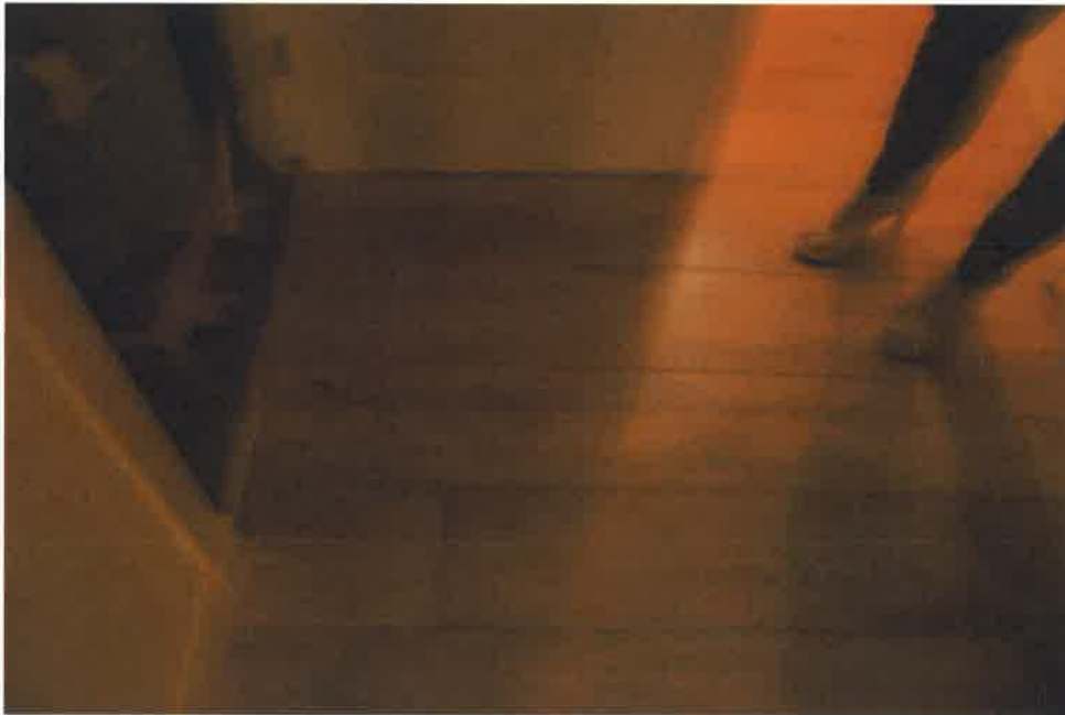
Floor of passage outside shower pump.
