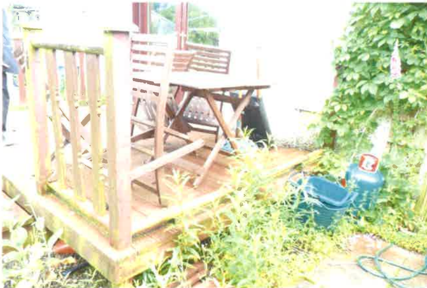
Patio fencing. Section removed on right hand side
