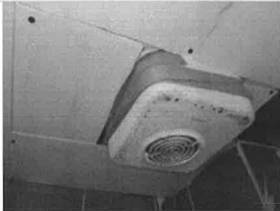
Bathroom Ceiling and extractor fan
