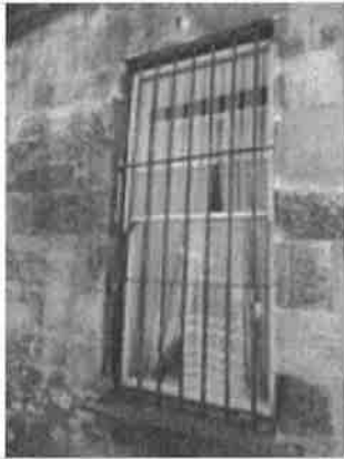
Rear window to back room
