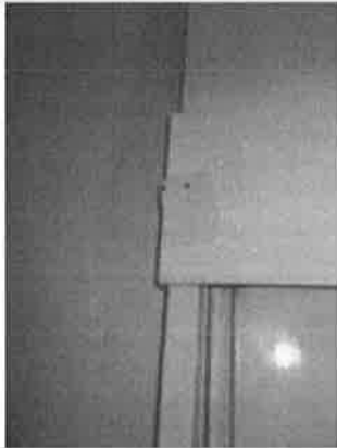
Back room - possible fitting for alarm
