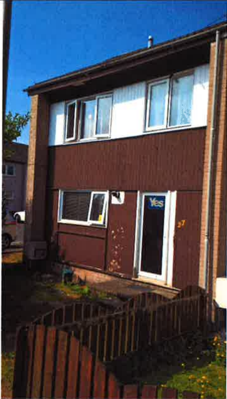
27 Cultrig Drive (Front Elevation). 2 bedroom, 2 storey, end terrace, brick house. Exterior in a poor state of repair.
