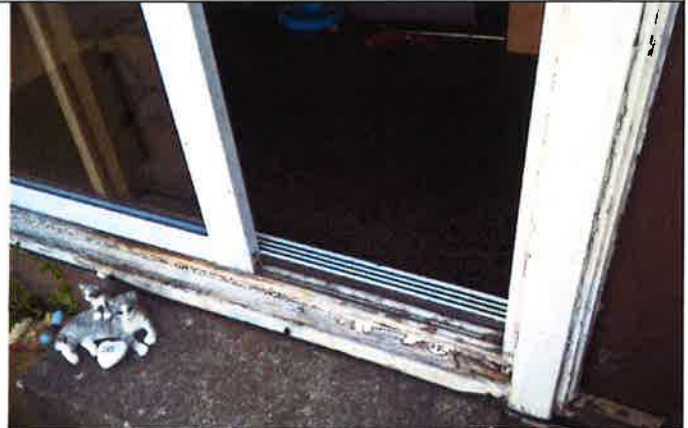
Close up of patio door.
