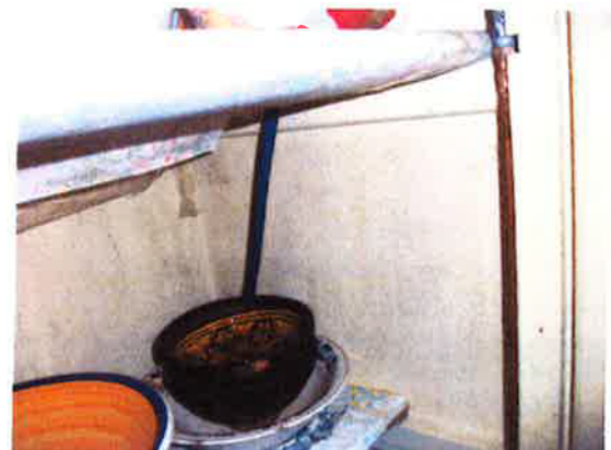
08 - Kitchen cupboard showing supply pipe
