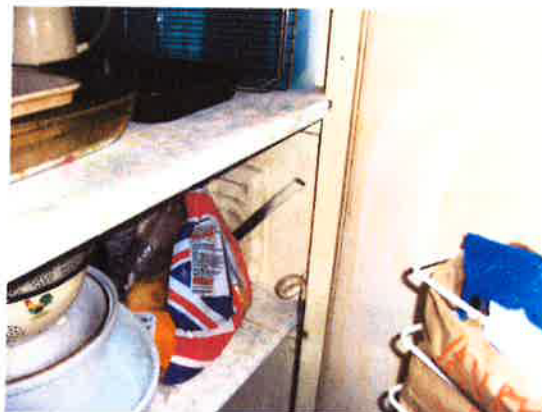
07 - Kitchen cupboard showing supply pipe
