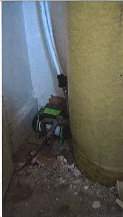
Pump fitted but pressure in shower is still poor. Flat undergoing complete renovation
