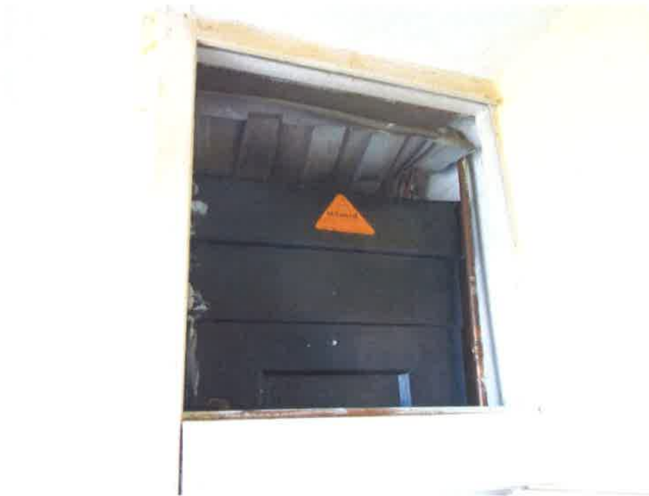
Cold water tank
