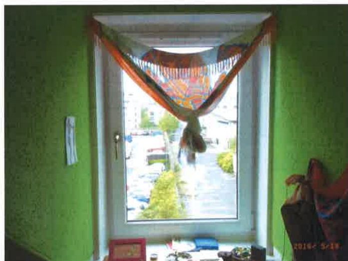
Replacement window in Bedroom
