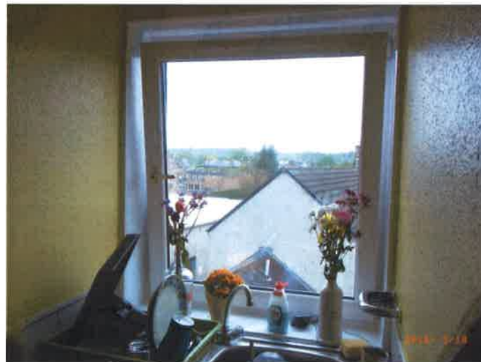
Replacement window in Kitchen
