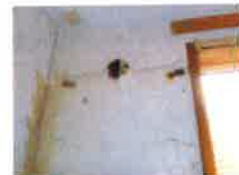
13. Hole For Former Flue Kitchen
