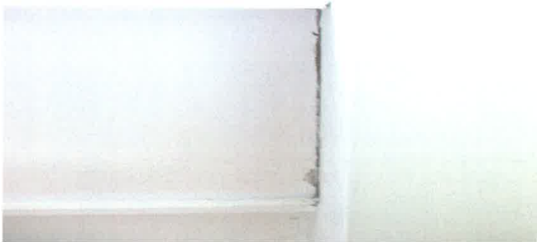
Bedroom 1 - Crack beneath right hand corner of window
