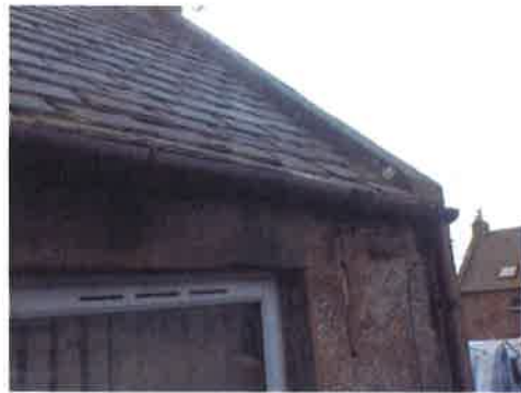
Roof above bedroom
