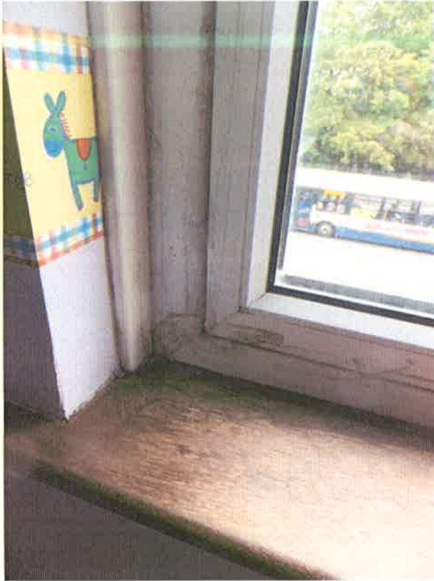
Window in upstairs bedroom
