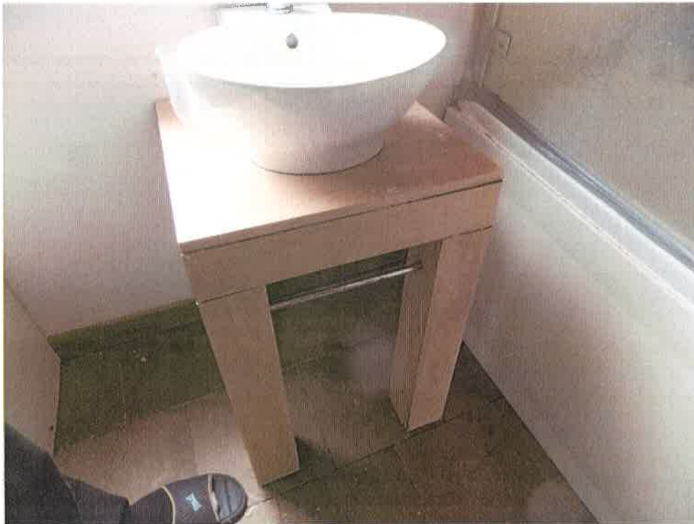
Sink in upstairs bathroom
