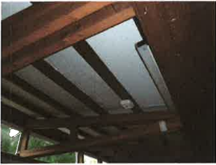
5. Ceiling/beams at open plan area
