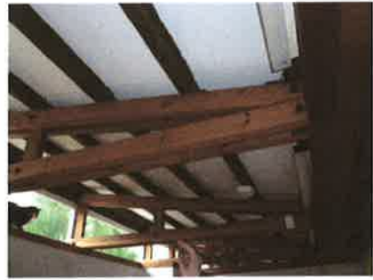
6. Ceiling/beams at open plan area
