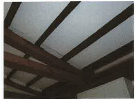
4. Ceiling/beams at open plan area
