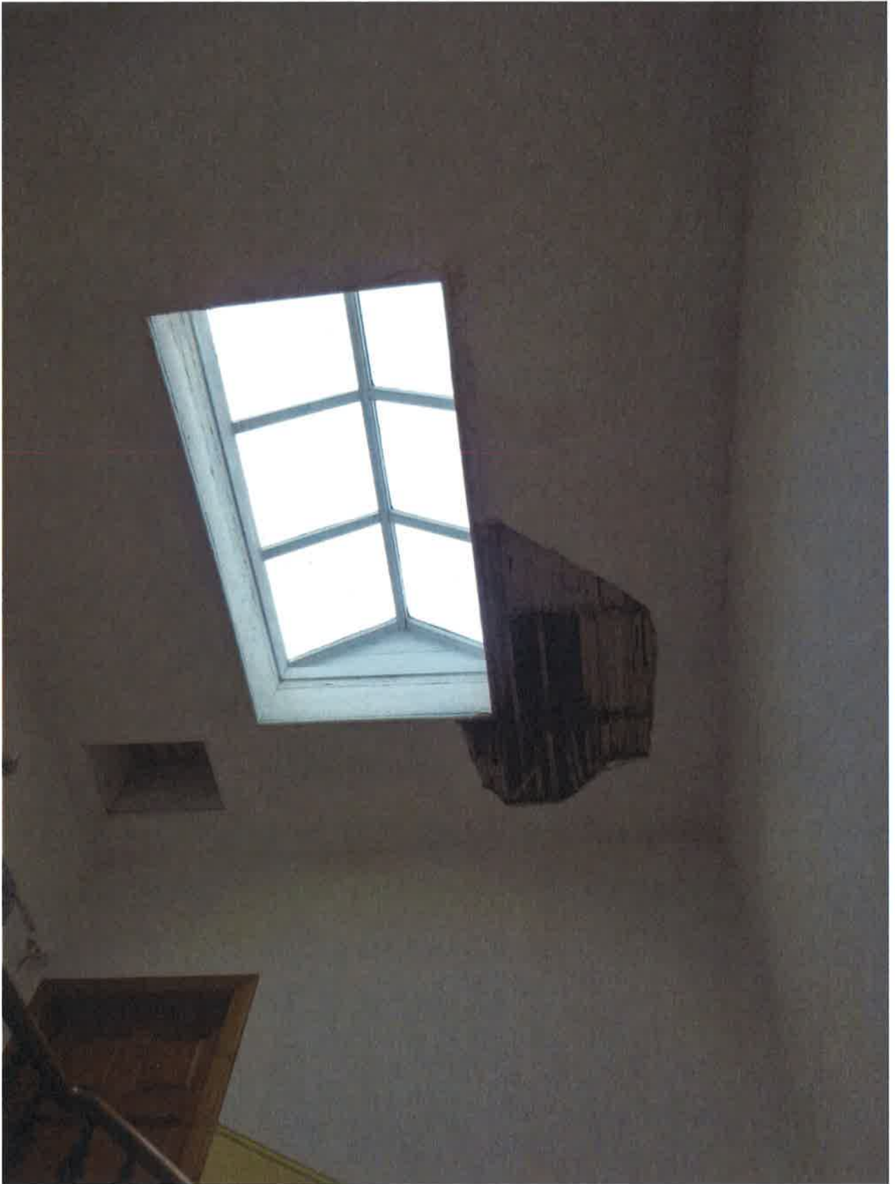
Leak around skylight
