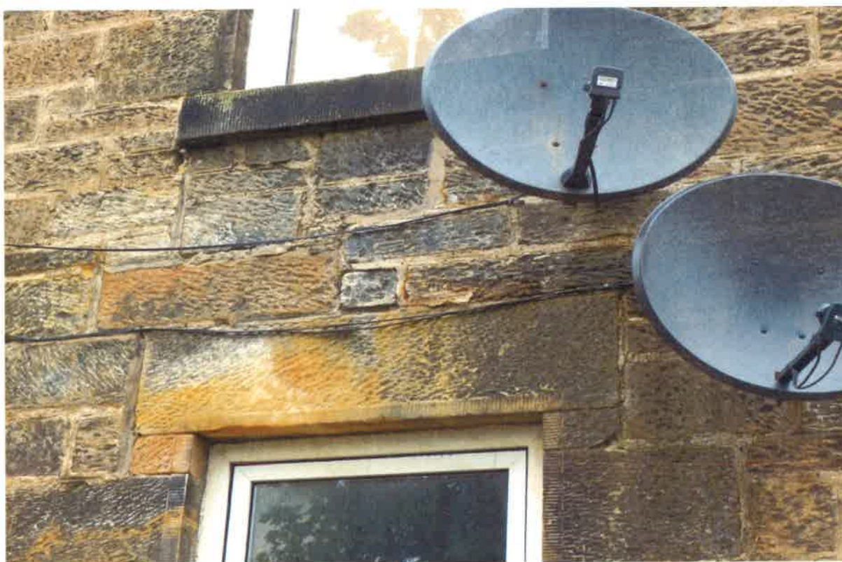
Eroded joints to front elevation
