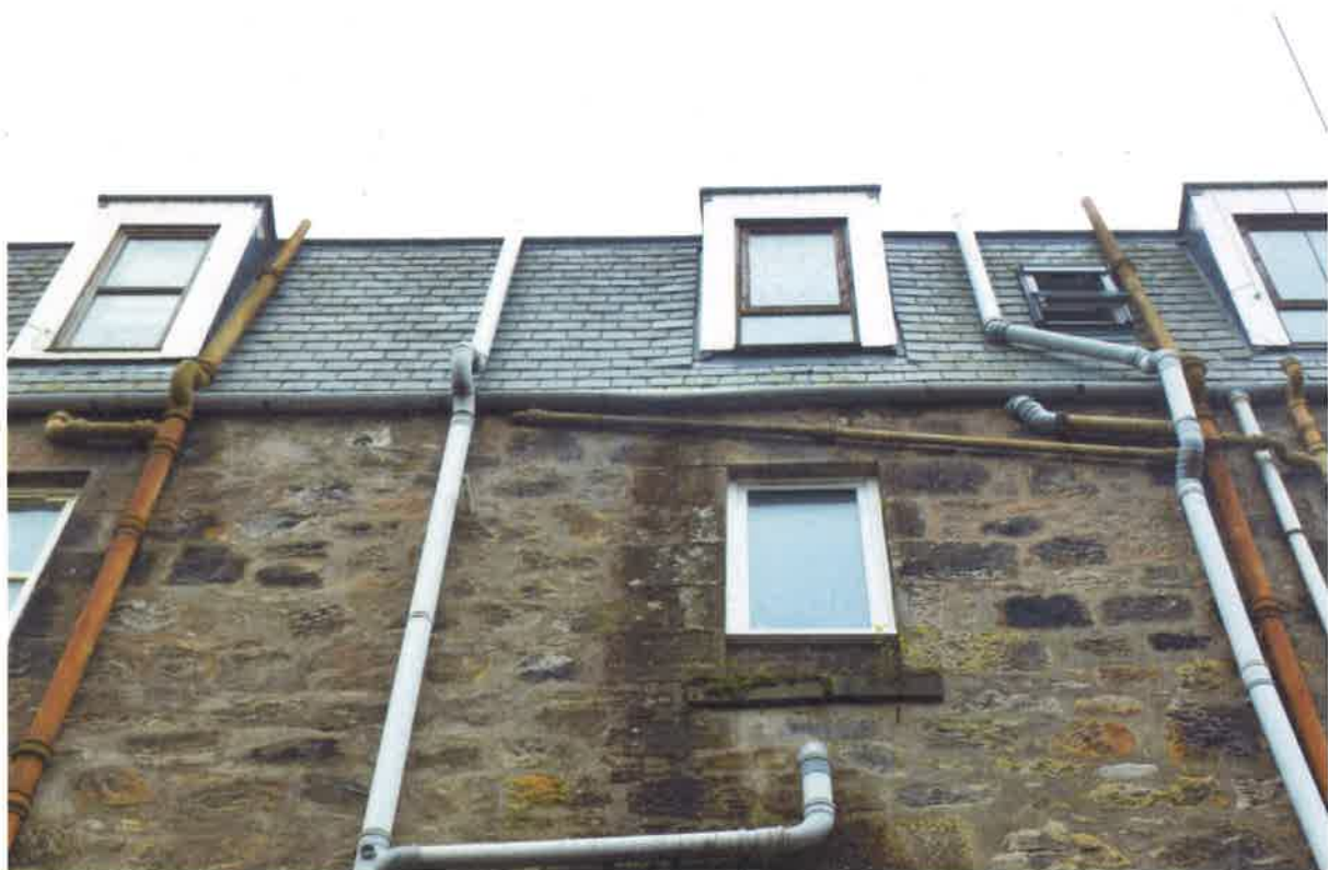
Rear gutters twisted
