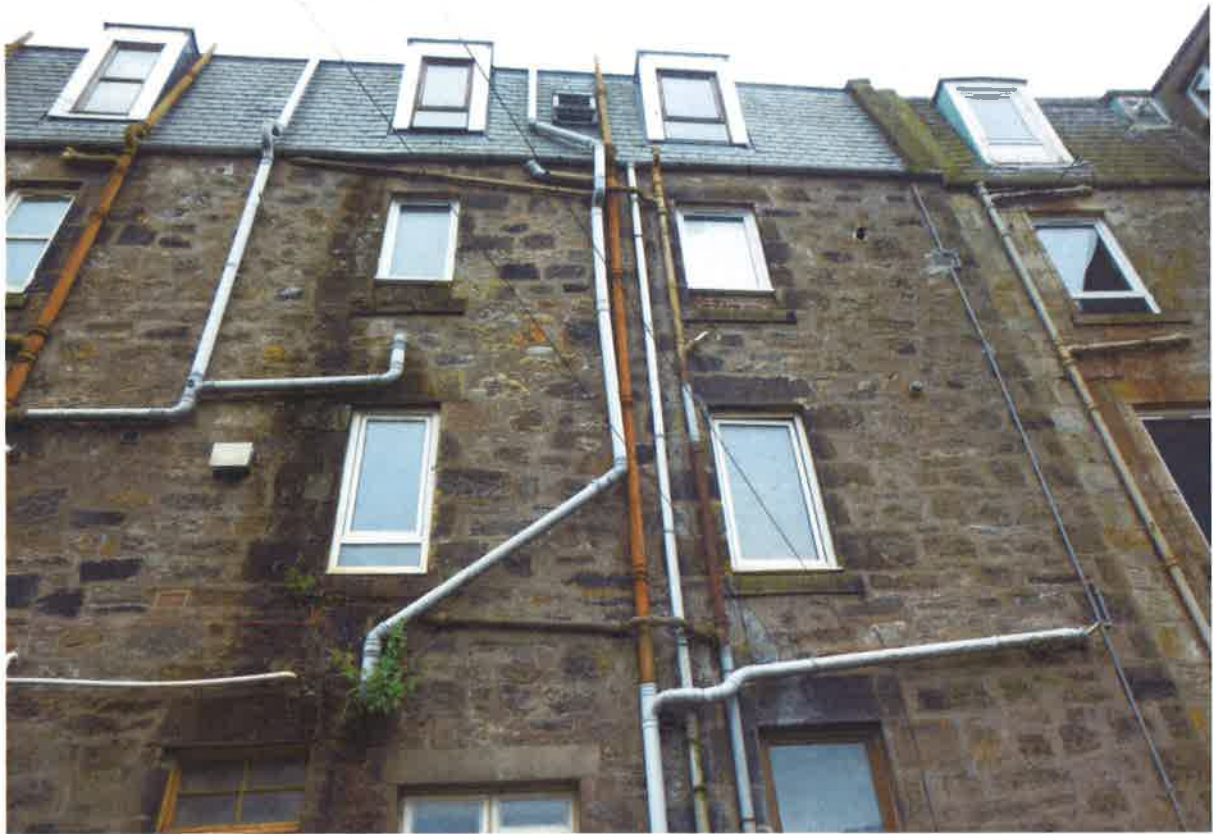
Rear elevation water damage
