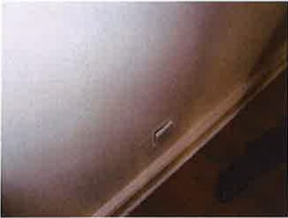
8. Living Room Electrical Socket
