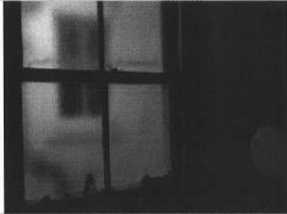
Main Bathroom - window onto light well
