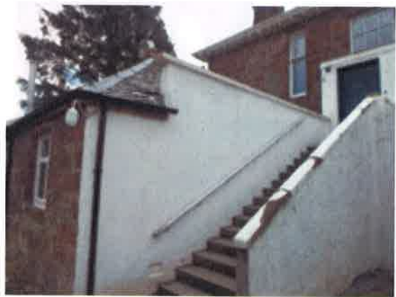
External rear single storey projection and access steps to upper flat
