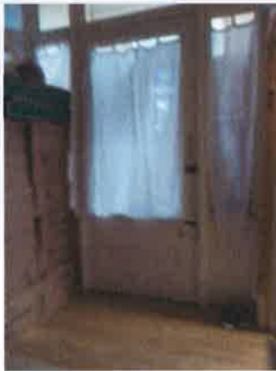
Front door - internal
