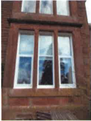
Living Room Window - External
