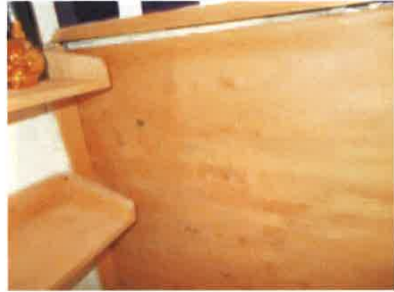
Main Bathroom behind toilet cistern
