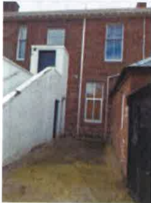
External down pipe to rear single storey projection
