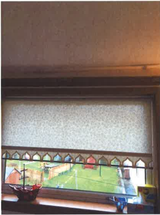
Photograph 7 : Showing black/grey mould above curtain rail
