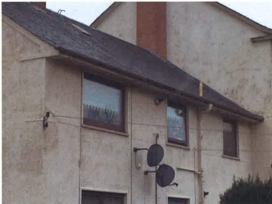
Photograph 2 : Rear elevation, gutters and roof
