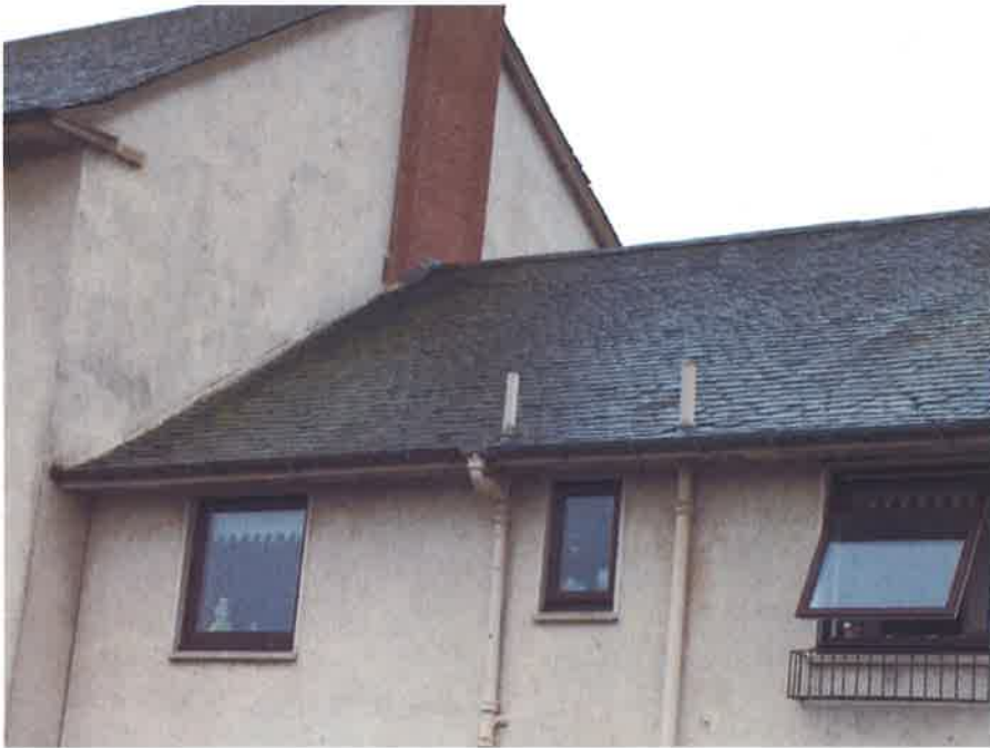
Photograph 1: Front elevation, gutters and roof
