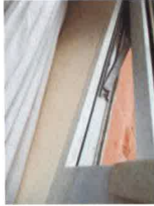
Front large bedroom window - left - lower section
