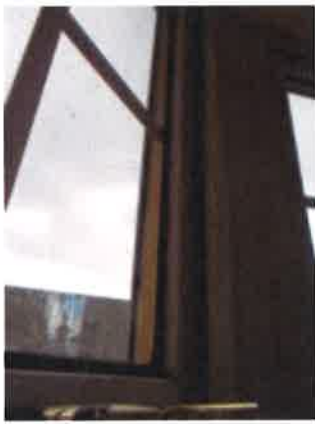
Front large bedroom window - left - lower section
