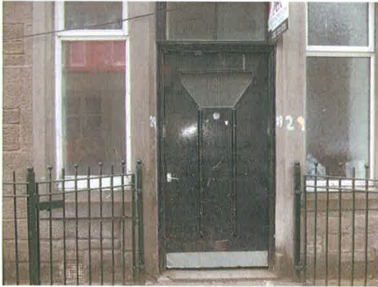
Communal Front Entrance Door (Externally)
