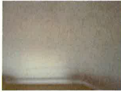
6. Small bedroom ceiling
