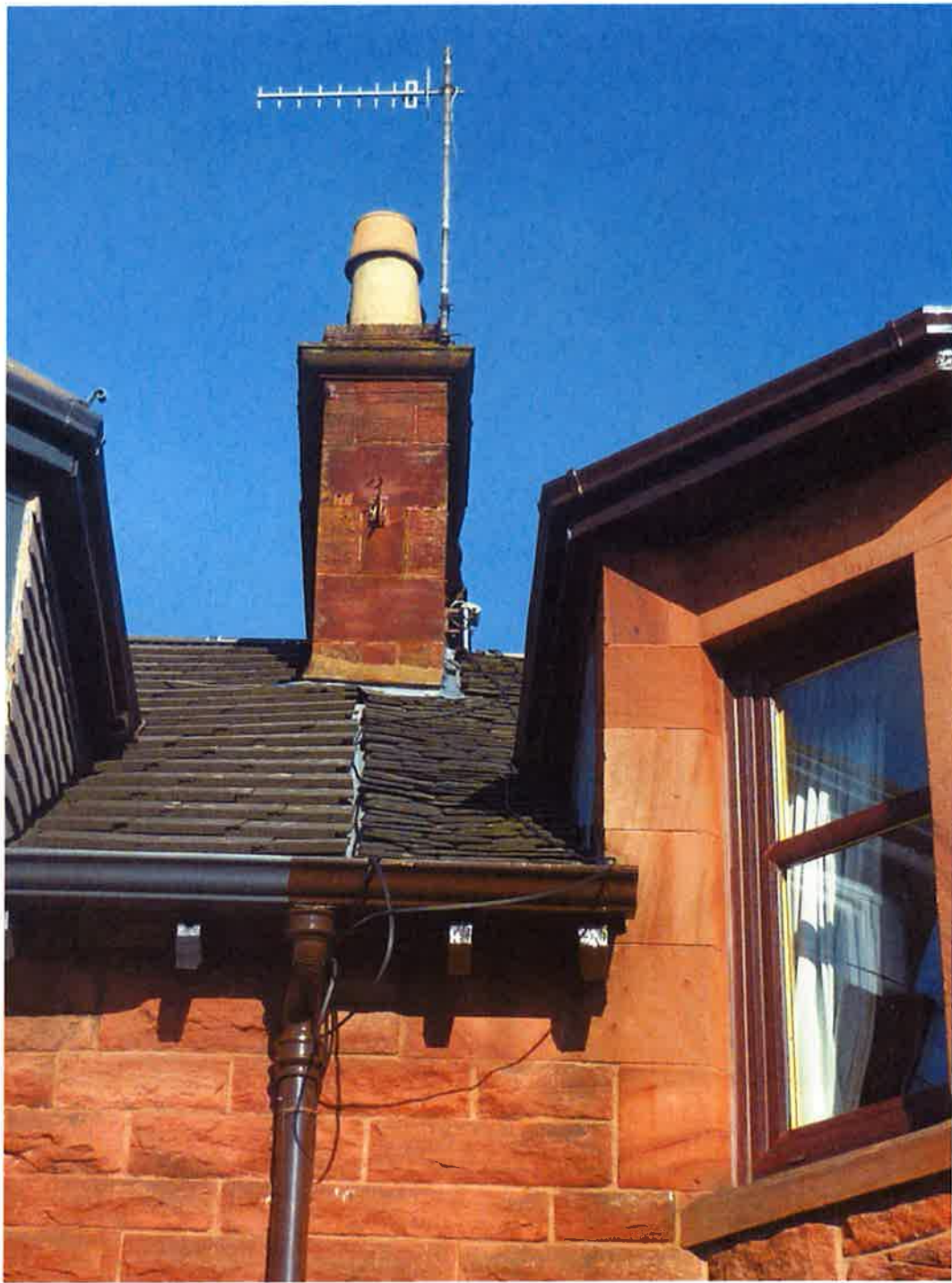
12. Detail - roof adjacent chimney and bay window
