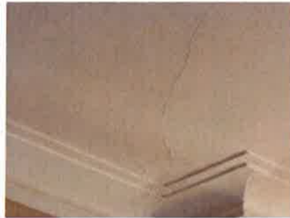
9. Main bedroom ceiling
