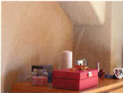
8. Main bedroom ceiling
