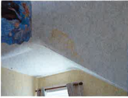
5. Small bedroom ceiling
