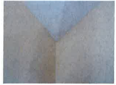
7. Small bedroom ceiling
