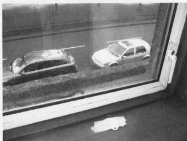
05- Front window showing condensation
