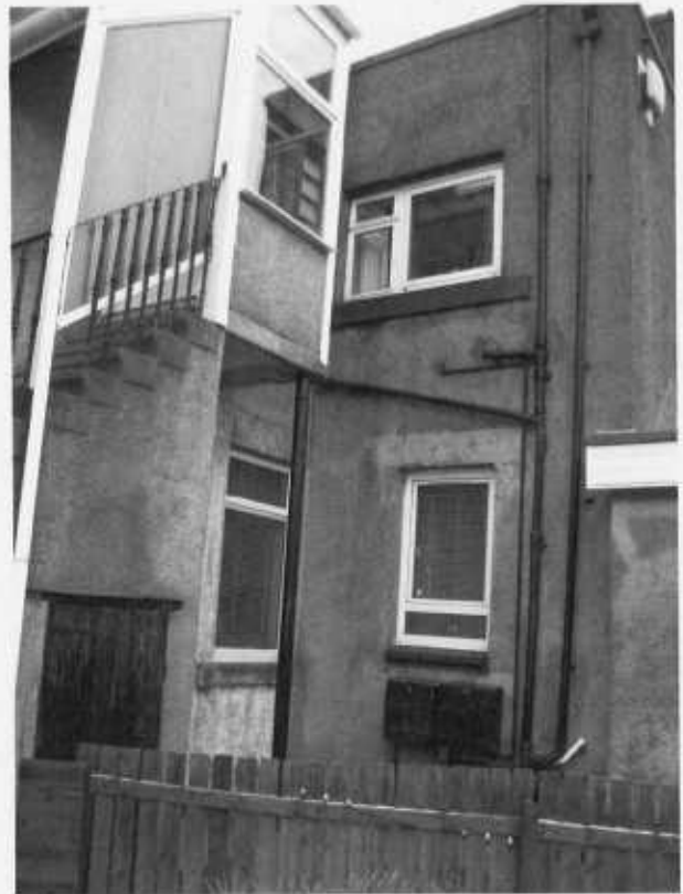
08 - Rear elevation, access & utility room
