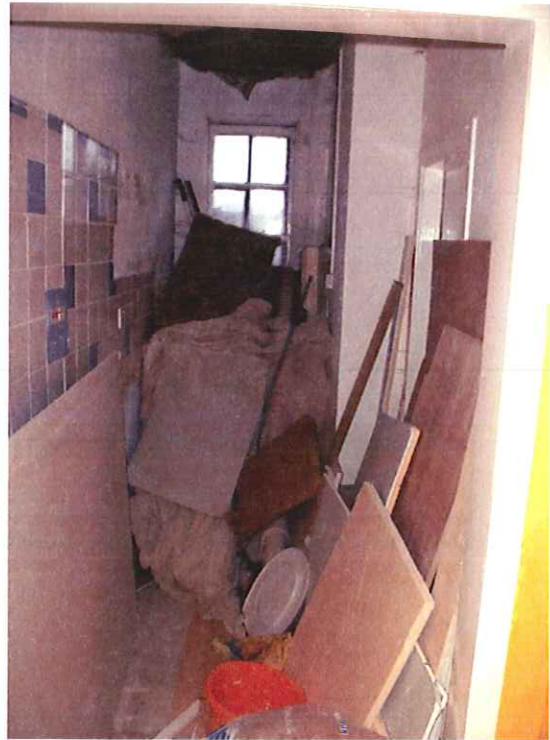
02 – Kitchen (as at Inspection)
