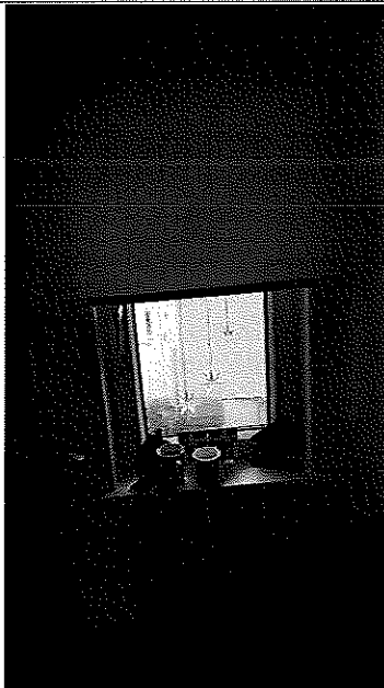
Stair window does not open or close
