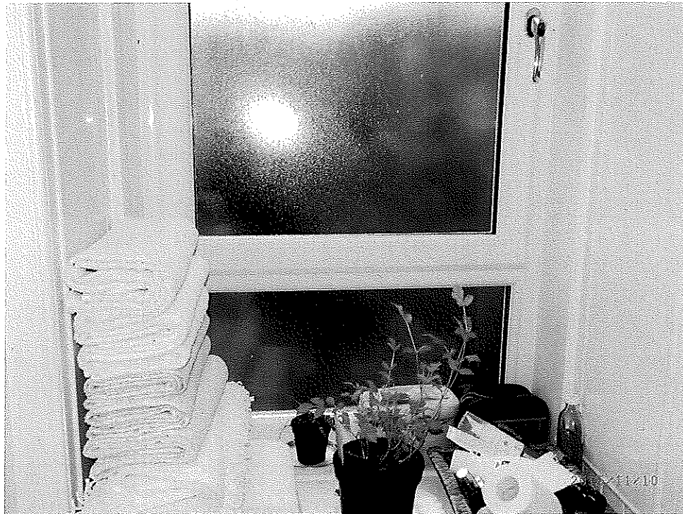
Bathroom replacement window
