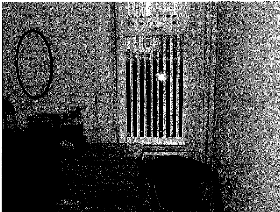
Bedroom replacement window/blinds
