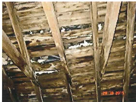
Attic-rear roof slope
