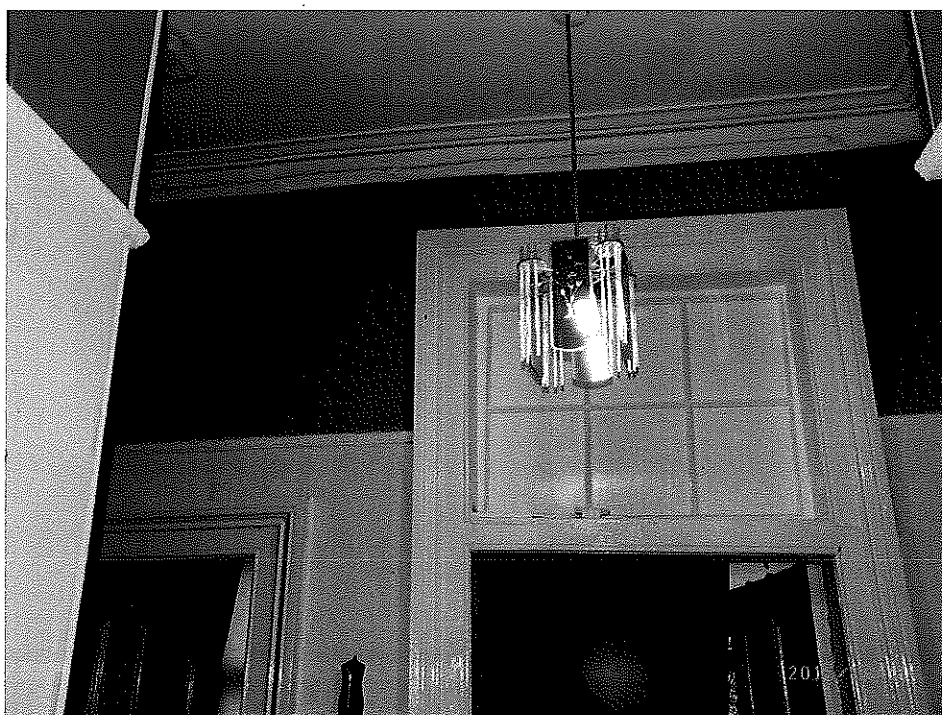
Drop in Bedroom door frame/cornice visible from Hall
