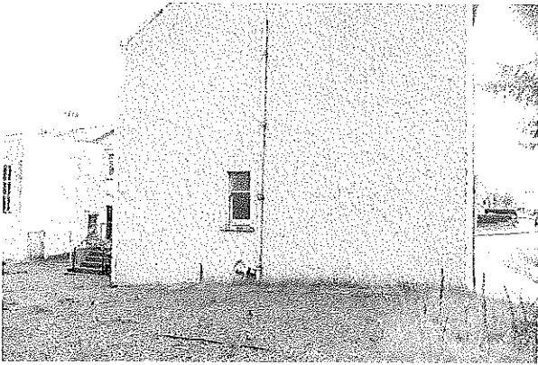
External view – bathroom window in gable wall
