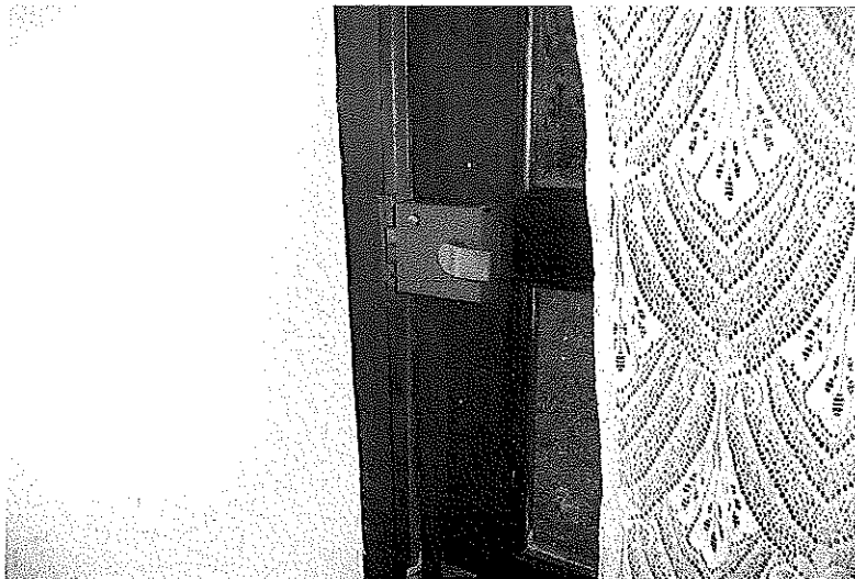
Front Door – Note missing snib staple / keeper
