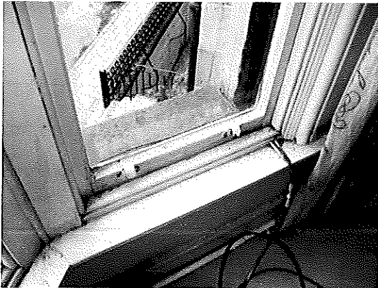
03 – Bay window (R) – showing repair
