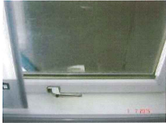
Upper Landing window - PHOTO 32
