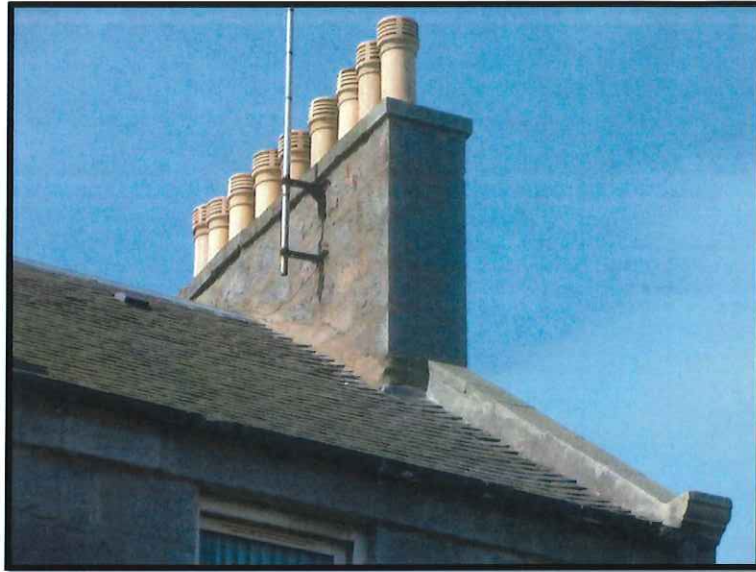
Figure 2 Front view West Chimney
