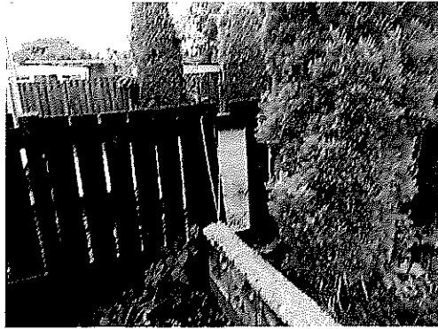
Rear Boundary fence
