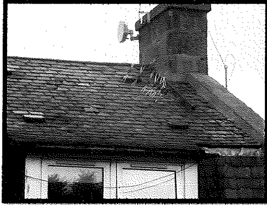
Figure 3 Rear Roof Slope
