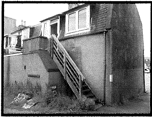
Figure 4 Rear Stair Overview
