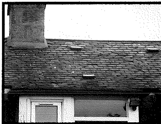
Figure 2 Rear Roof Slope
